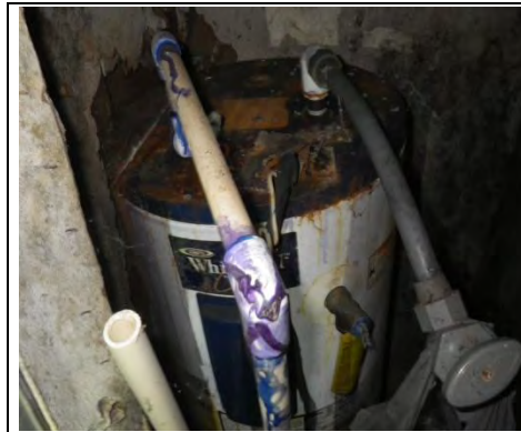
water heater is very old with improper wiring
