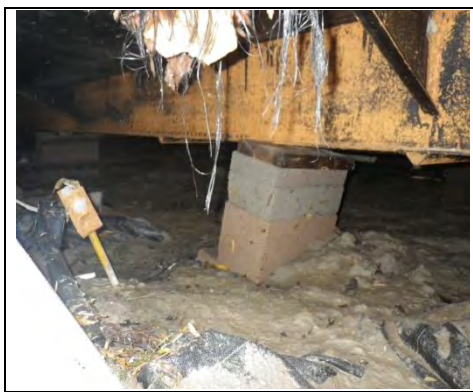
Missing tie down and damaged insulation
