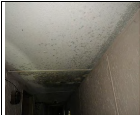
Water stain and mold on ceiling
