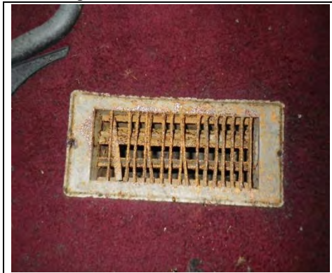
Rusted floor duct
