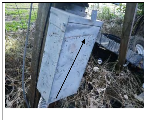
water mark on exterior disconnect
